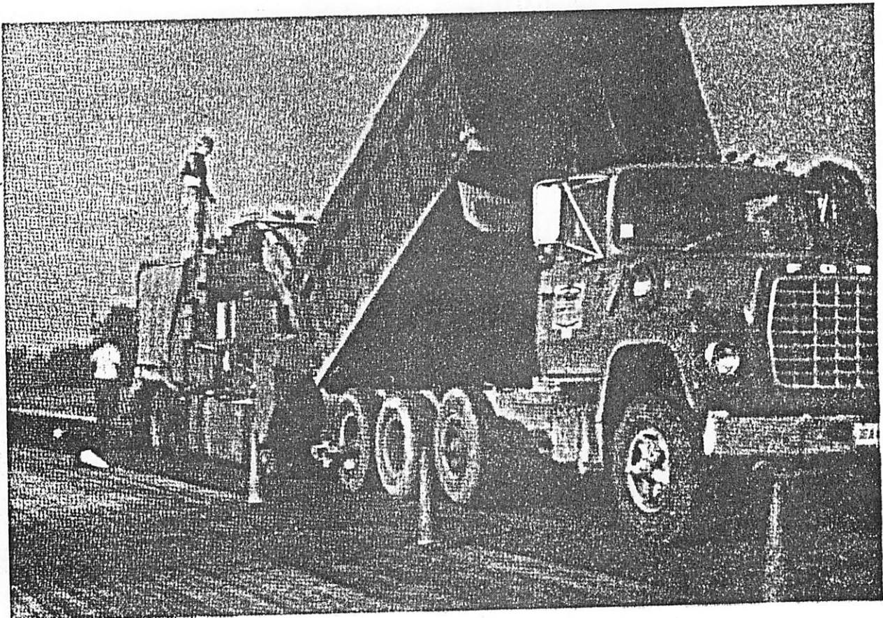
Self-propelled continuous slurry machine applying ODOT type C slurry to Ohio SR 42 near Xenia. Late August - 1977.
